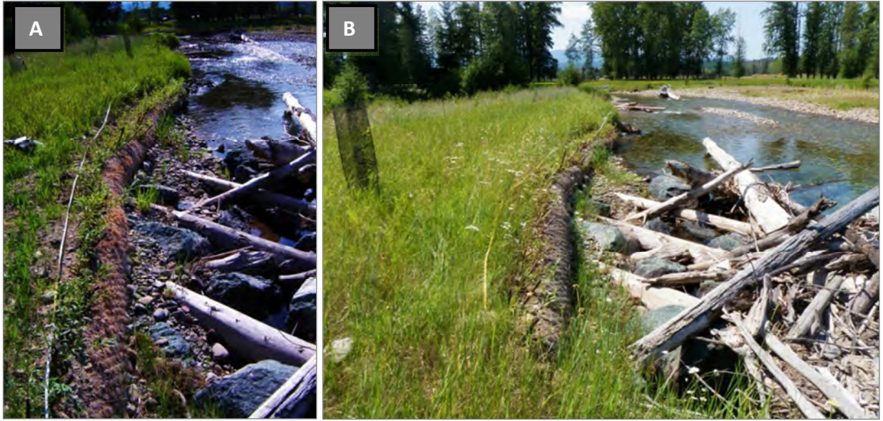
Figure 4-12. Photographs of Coir Log 12 (installed in 2008) in 2009 (A) and in 2010 (B).
