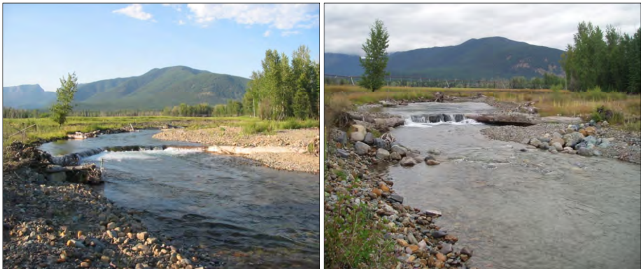
Figure 2-4. Photos of Phase 1 in 2004 (left) and 2009 (right). A log cross vane built to maintain vertical grade control at the pool tailout is visible in the photos.
