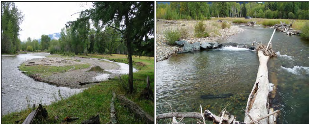
Figure 2-8. Photos of the pool cross-section at Station 19+25 ft in 2001 (left) and 2010 (right).
